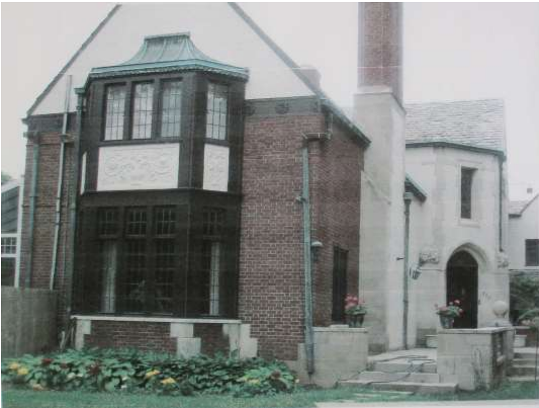
An undated photo of 315 Lakeland Street. Photo courtesy of the Grosse Pointe Historical Society.
